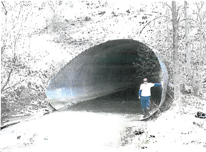
Photo 11 - Dochart Creek - 7,620 mm X 4,240 mm SPCSPA at Cambell Drive
