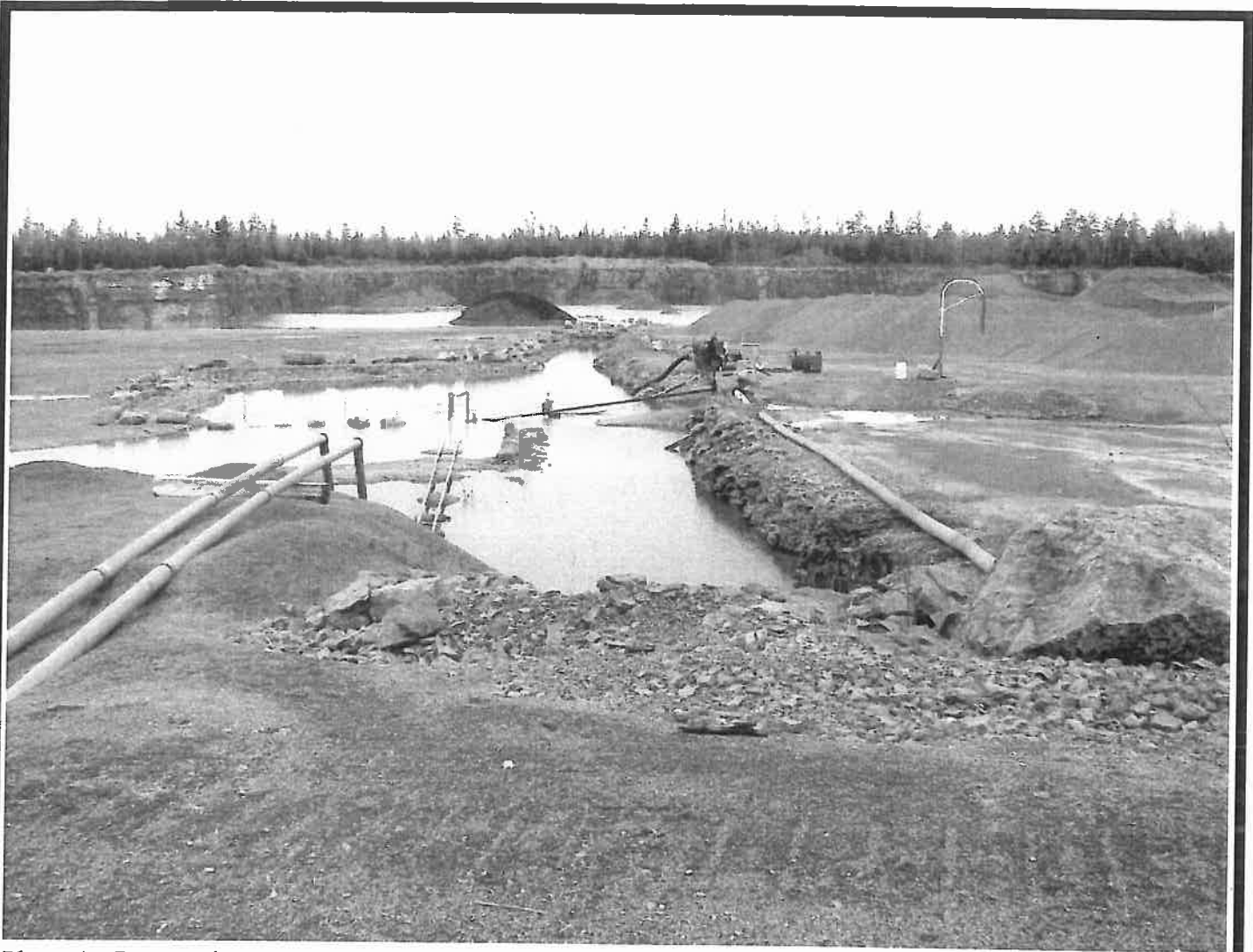
Photo 1 - Dewatering Operation
