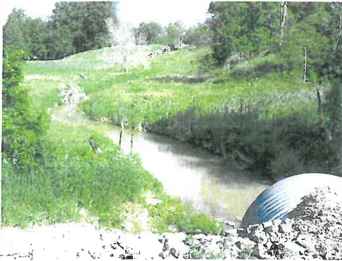
Photo 12 - Ryan Creek looking upstream of 2,740 mm Dia SPCSP at Carmichael Sideroad
