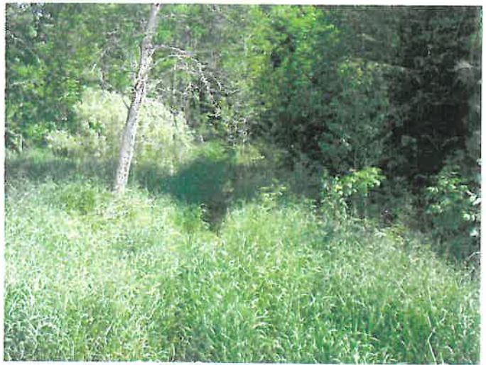
Photo 14 - Unnamed Drain looking upstream of 600 mm Dia CSP at Golf Club Road
