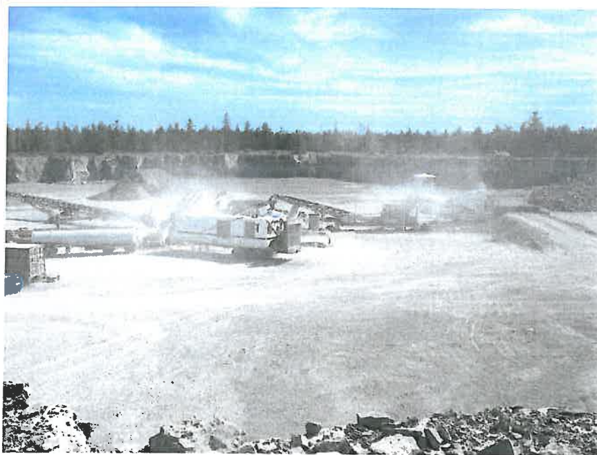
Photo 17 - Aggregate Production and Rock Drilling
