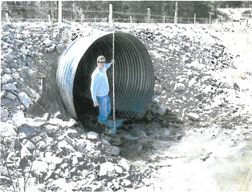
Photo 10 - Ryan Creek 2,740mm Dia SPCSP at Carmichael Sideroad
