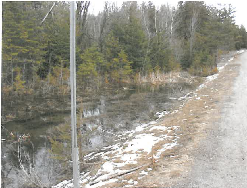
Photo 18 - Usborne Street Roadside Ditch looking southeast from "T" intersection with Campbell Drive.
