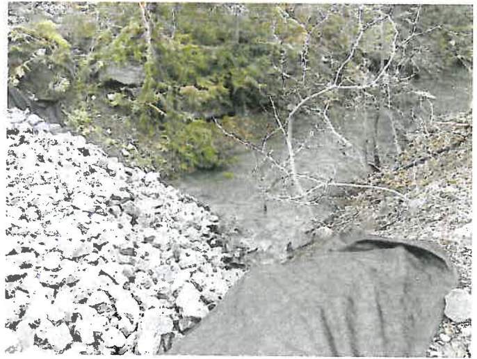
Photo 4 - Outlet Channel immediately downstream of Sediment Basin
