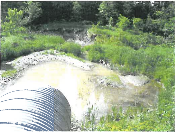
Photo 13 - Ryan Creek looking downstream of 2,740 mm Dia SPCSP at Carmichael Sideroad
