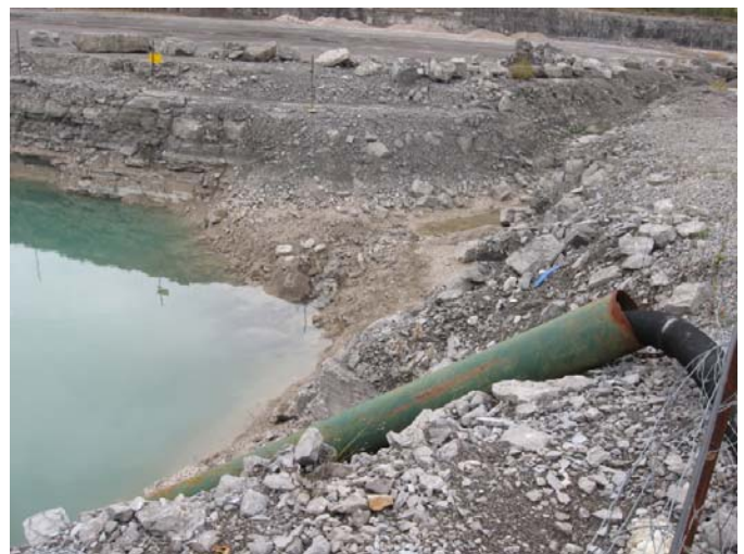
Photo 22: October 14, 2009 – note the sump level is below the base of the floor ditch
