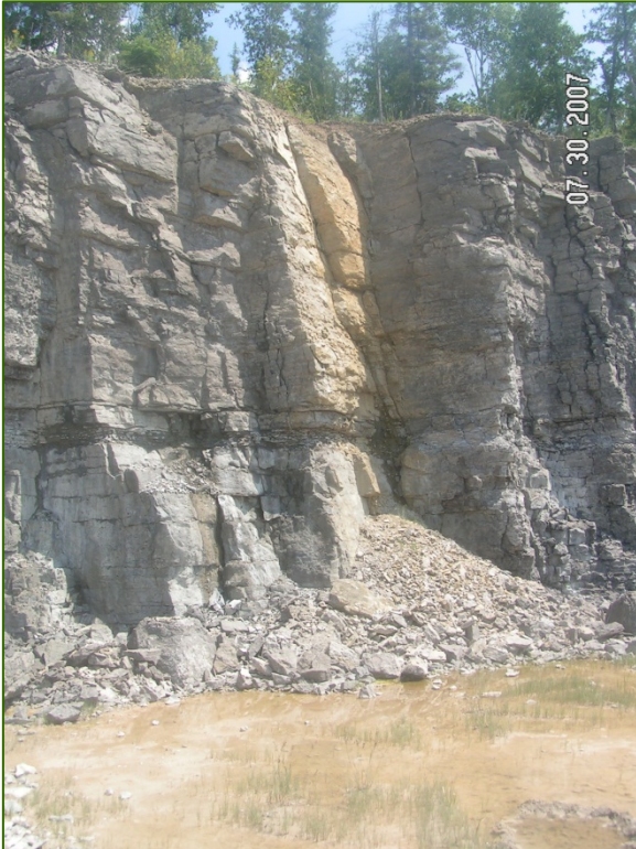
Photo 4: Iron staining on face shows how surface water migrates down to significant levels – note minor seepage from lower 3 m.
