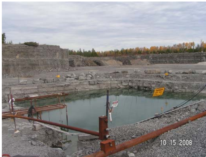
Existing ("Main") Sump -2009
