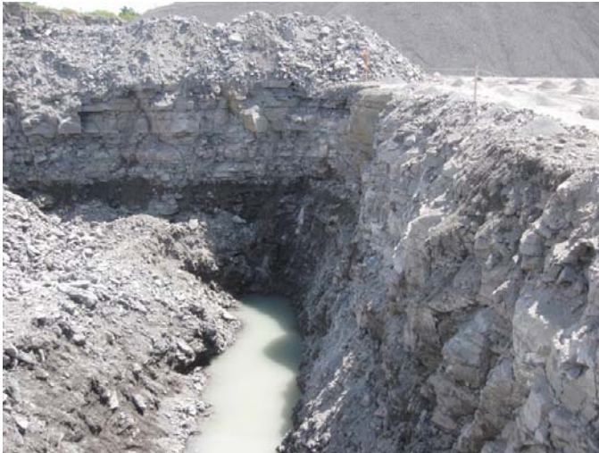
Photo 23: After initial blast, August 12 2009. Face shows dampness below K-bentonite layer probably due to disturbance during blast
