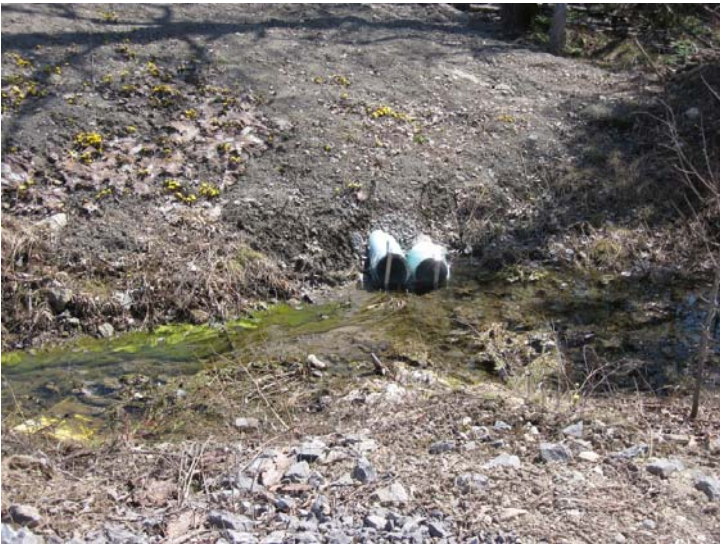
Photo 10: Infiltration Drains around home in Ridge View Estates, typical
