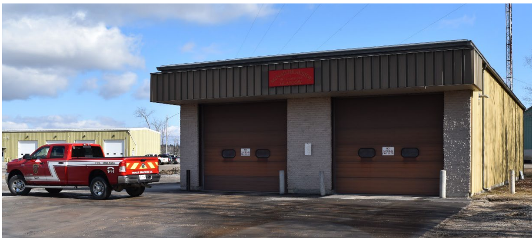
Figure 5. Exterior of Fire Station 1 – Glasgow.
