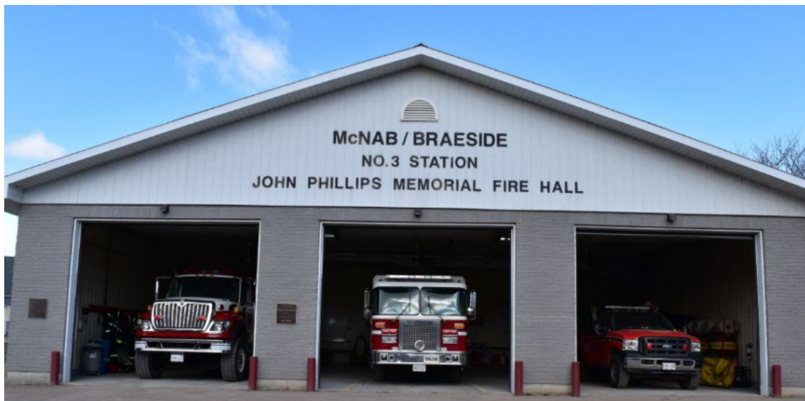
Figure 9. Exterior of Fire Station 3 – Braeside.
