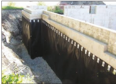
A gap around the basement wall in a home that is under construction.
